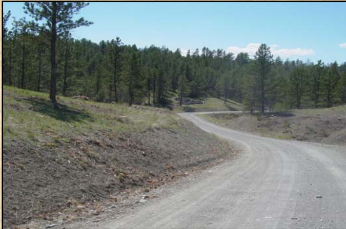
Owl Canyon Right-of-Way Ingress/Egress Clearing Project
